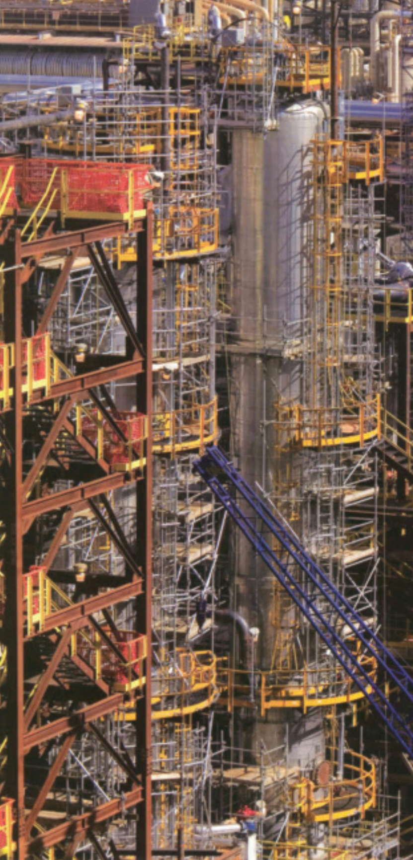
Fig. 1 — The cylindrical tower of a typical coker.
