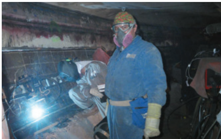
Fig. 3 — Nine-ft-wide windows were cut out of the inner skirt to allow access to the corroded steel shell.
