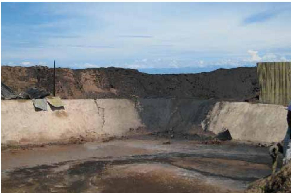
**Photo 6: the damaged flare pit following the Kingfisher-1 well test, showing damaged steel sheets**
