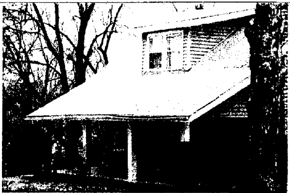
12. 7130 Virginia – Deteriorating roof.
