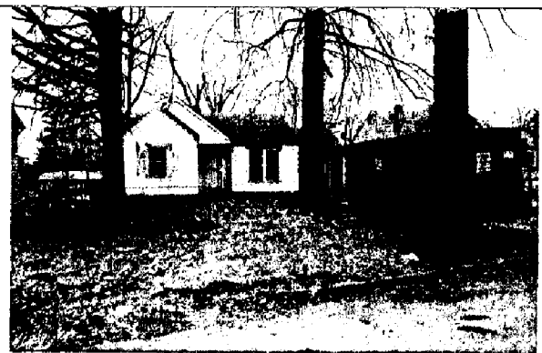
17. 7424 Park – Deterioration of house and dumpster in front yard.
