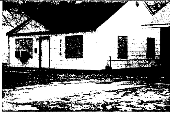
7. 7116 Wayne-Boarded up home.
