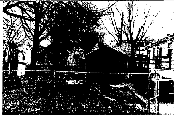
8. 1800 72 nd Street- Lacks garage or carport, unfinished remodeling on back porch.
