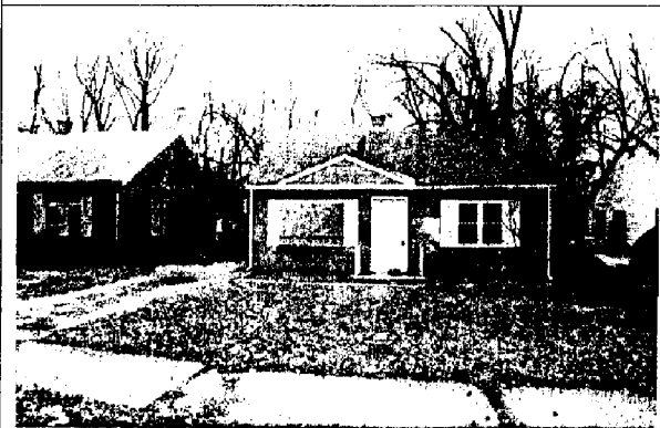
5. 7108 Wayne- Vacant home and deteriorating driveway.
