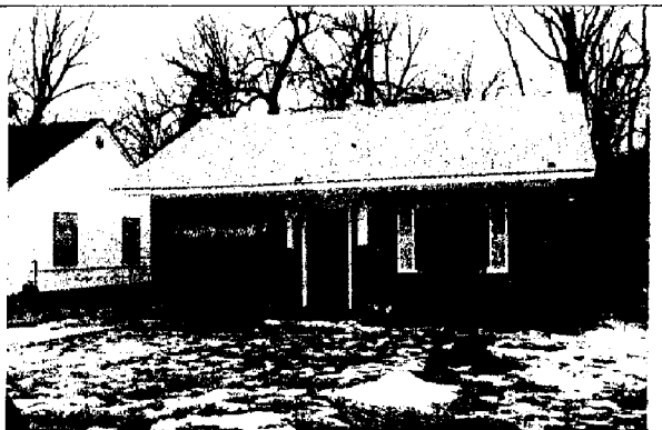
6. 7112 Wayne-Boarded up and vacant home.
