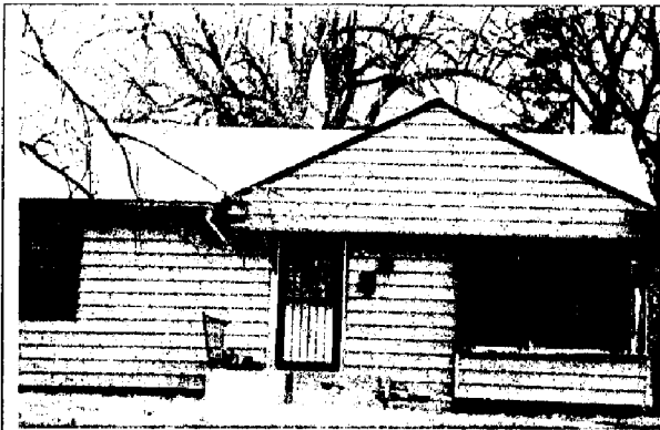
13. 7444 Tracy - Guttering falling off house and porch steps deteriorating.
