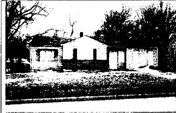
1. 1115 E. Gregory Blvd- Vacant and boarded up home.
