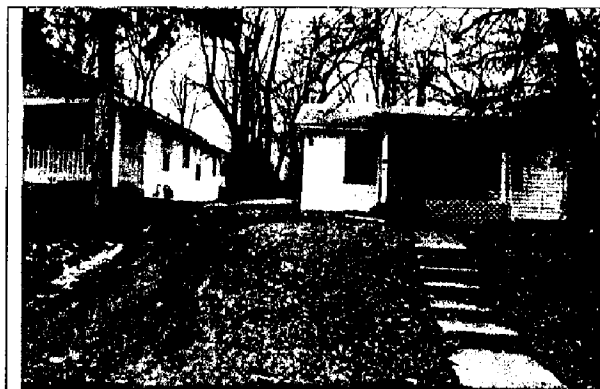
19. 7102 Wabash – Dirt driveway and no sidewalk.
