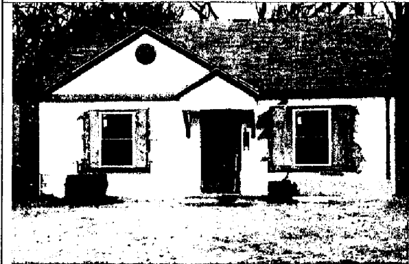
3. 1506 72 nd Street- Unfinished renovation of exterior.
