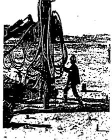
Superior Blasting drilled 3-inch diameter blast holes 17 - 20 feet deep on 3 x 3 pattern with 1-R track drift.
