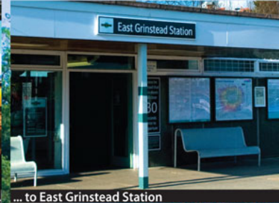
... to East Grinstead Station
