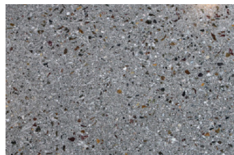
Fine aggregate or salt & pepper finish - remove not more than 1/16"
