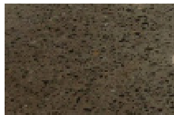
Medium aggregate - remove not more than 1/8"
