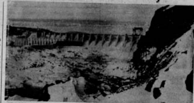
The Shipshaw hydro-electric development is nearing completion in the wilds of Northern Quebec to supply power for Aluminum, Ltd., of Canada. The Chute a Caron powerhouse and dam are shown.
