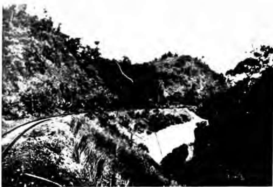
VIEW OF REGRADED TRACK AT THE BAHIA BUAYA GORGE, MAIN LINE SOUTH SHOWING A PORTION OF REMAINING WALL
