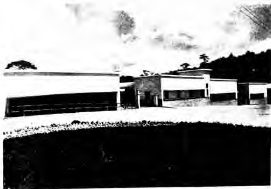
NEW GARAGE AND SHOPS OF THE BENGUET AUTO LINE, BAGUIO.
