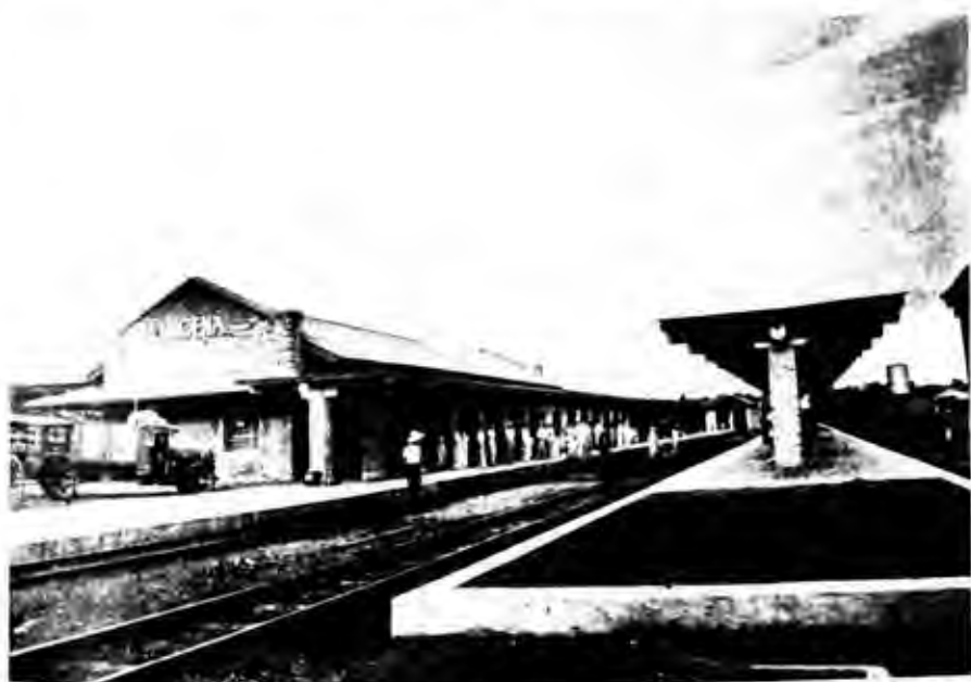
NEW STATION AT LUCENA, TAYABAS, SHOWING ISLAND PLATFORM WITH PASSENGER SHELTERS.
