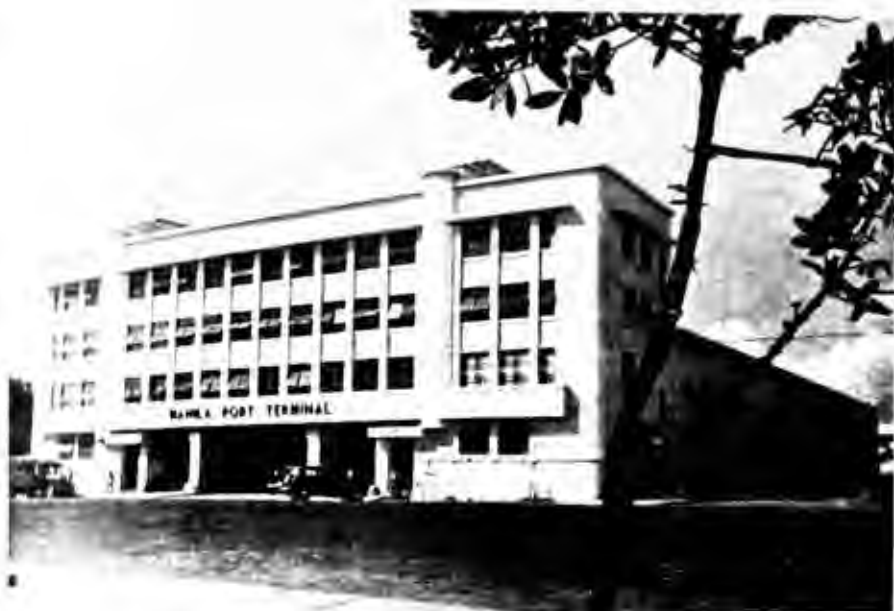
NEW MANDA PORT TERMINAL BUILDING OPPOSITE PIER 7, PORT AREA.
