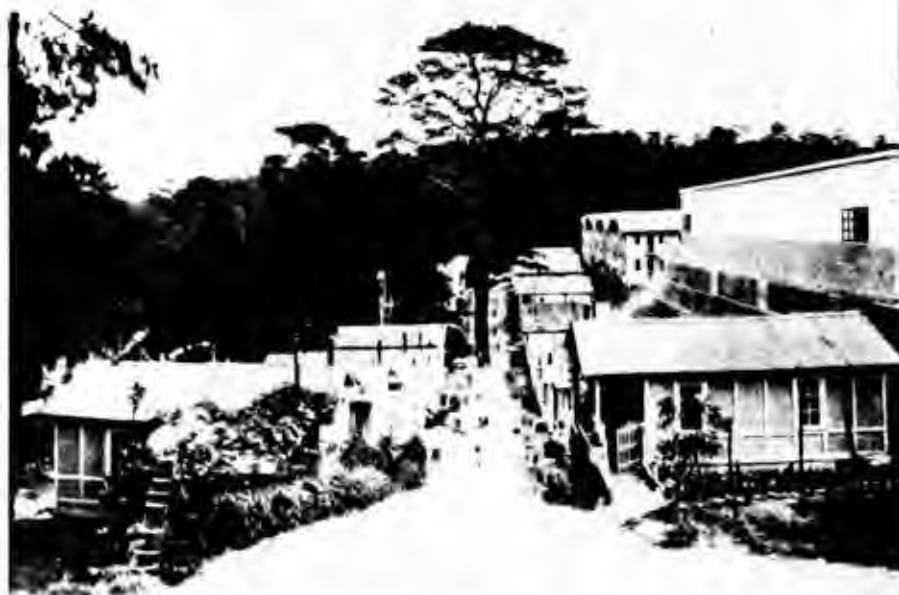
VIEW SHOWING NEW COTTAGES CONSTRUCTED FOR EMPLOYEES OF THE BENGUET AUTO LINE AND THEIR FAMILIES AT REAR OF NEW SHOPS AND GARAGE IN BAGUIO.
