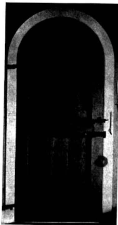
Fig. 13. Here is a Modern Adaptation of the Hand Forged Iron Strap Hinges, Latch and Bolt, Used on the Entrance of a Cottage at Woodstock, N. Y.
