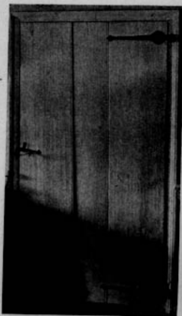
Fig. 4. A Batten Door in the Old Van Buren House, Kingston, N. Y., Showing the Use of Strap Hinges and Latch.
