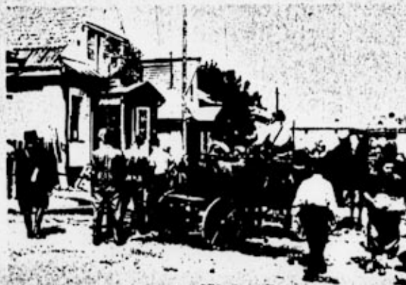
Primitive fire-fighting apparatus - Water had to be carried from the nearby river in barrels and hand-pumped. The incendiary bombs dropped by the German planes caused considerable fire loss to residential and business properties.
