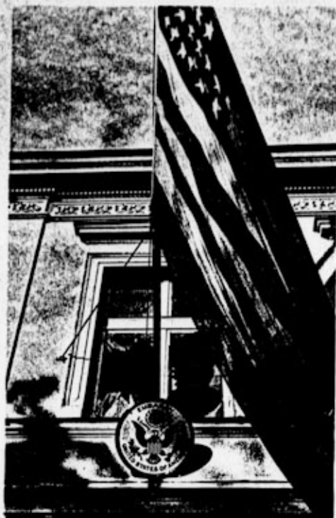
After the first week of the war - American Embassy in Warsaw struck by flying splinters of shells.
