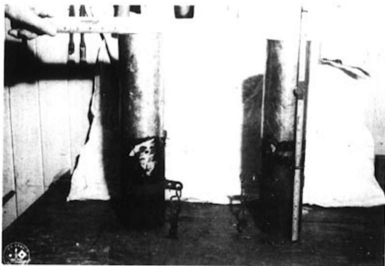
Figure 9 Two of four incendiary bombs found near Hayfork, California. Shows general appearance and "T" shaped objects which suspended the bombs from the periphery of the weight release mechanism.
