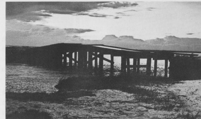
CHAPPAQUIDDICK ISLAND DYKE BRIDGE: Would be conserved and preserved by Kennedy legislation.
