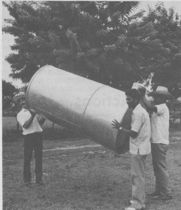
Agronomist Gary Reusche and Haitian agricultural technicians set up a model corn silo, which Mr. Reusche hopes will catch on with Haitian farmers. The silos are inexpensive and easy to fabricate.
