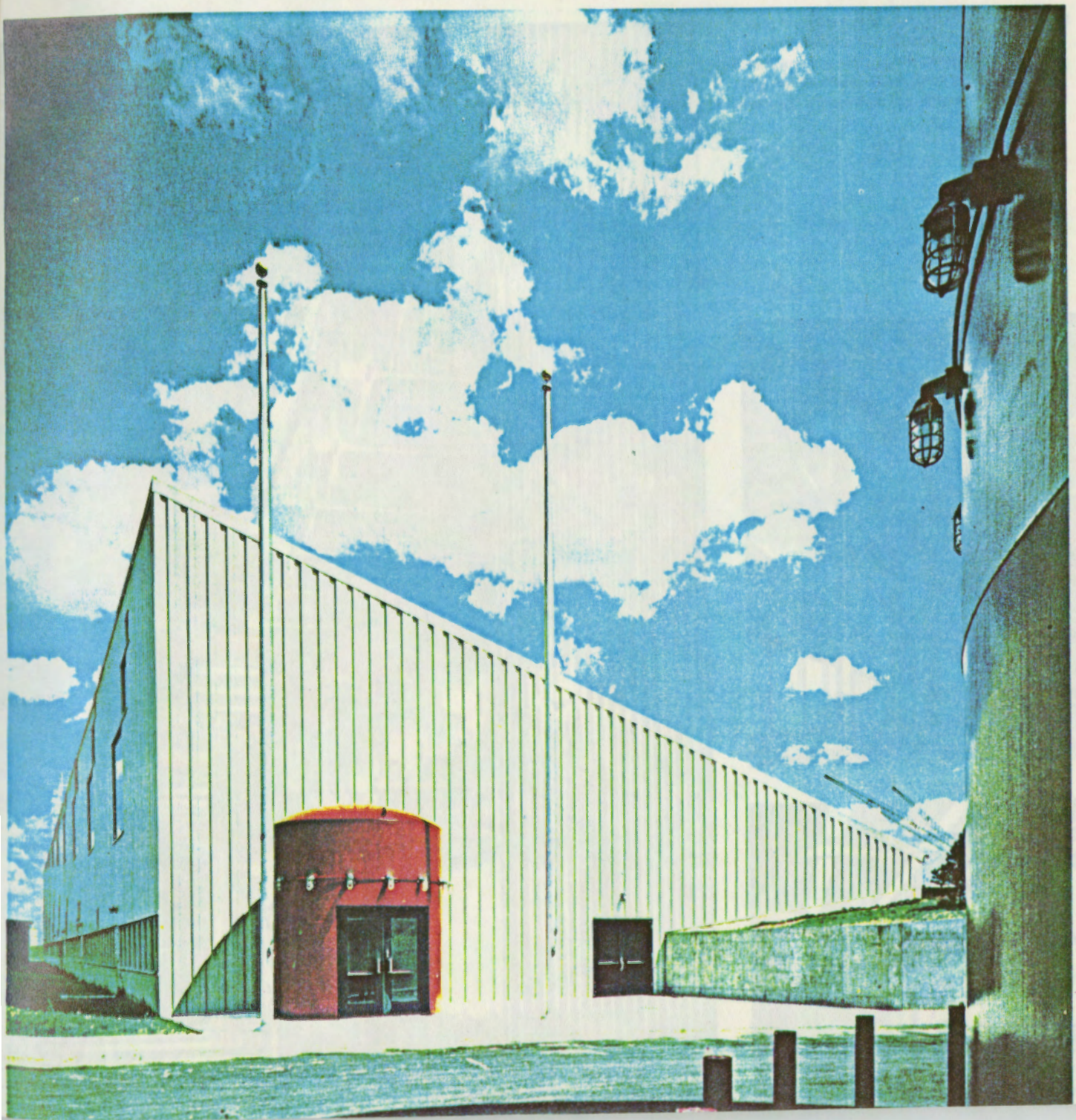
The corrugated metal administration and education building (this page and facing page top) is entered by sewer ducts through bermed earth.
