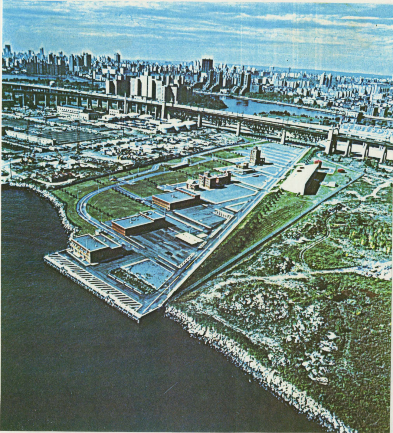
THE WARDS ISLAND TRAINING CENTER IS READY FOR IMMEDIATE OCCUPANCY BY THE NATIONAL FIRE ACADEMY
