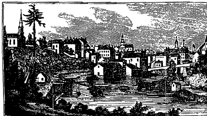
East View of Seneca Falls Village
