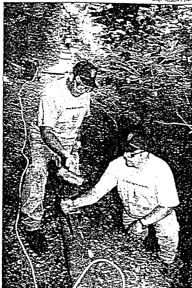
PATH TO SERVICE: Maryland Conservation Corps members Scott Walker (l.) and Kevin Walker repair trails along the Potomac River near Washington. Such volunteerism is growing.
