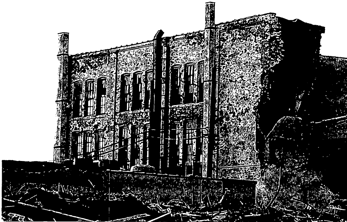
Demolition of dilapidated properties in the North of Main area of the city of Benton Harbor. Site for the new Atlantic Automotive Components Ox Creek Plant.
