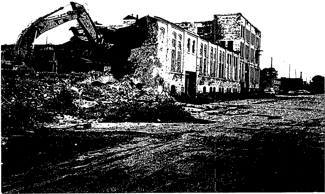
Demolition of dilapidated properties in the North of Main area of the city of Benton Harbor. Site for the new Atlantic Automotive Components Ox Creek Plant.
