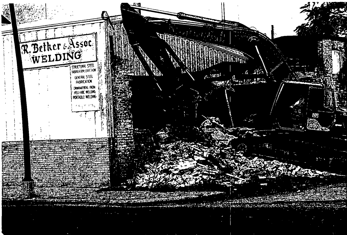
Demolition of dilapidated properties in the North of Main area of the city of Benton Harbor. Site for the new Atlantic Automotive Components Ox Creek Plant.
