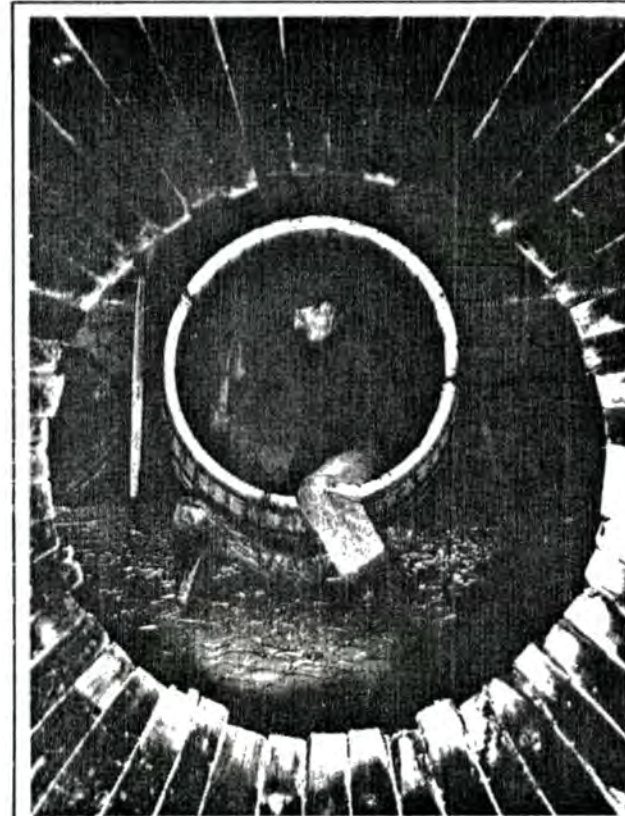
An Italian barrel maker works on a large wine cask, climbing inside to smooth the wooden staves. Constructed just outside Rome, the cask will later be filled with wine from the famous town of Frascati.
