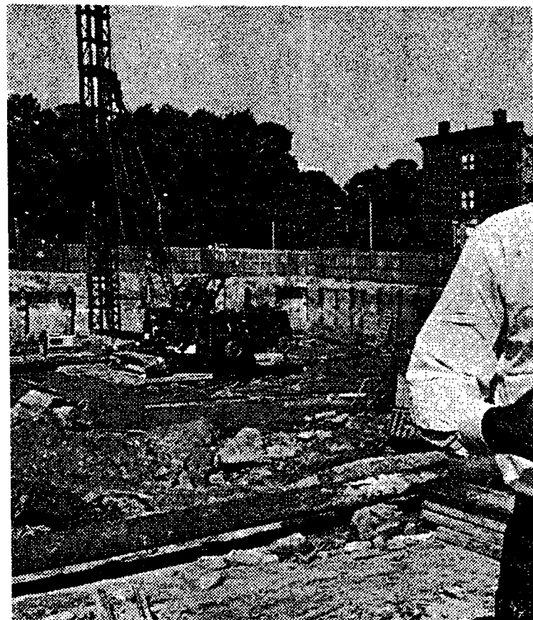
North General Hospital in Harlem has begun a $150 million rebuilding program that will make it the largest private development in the
