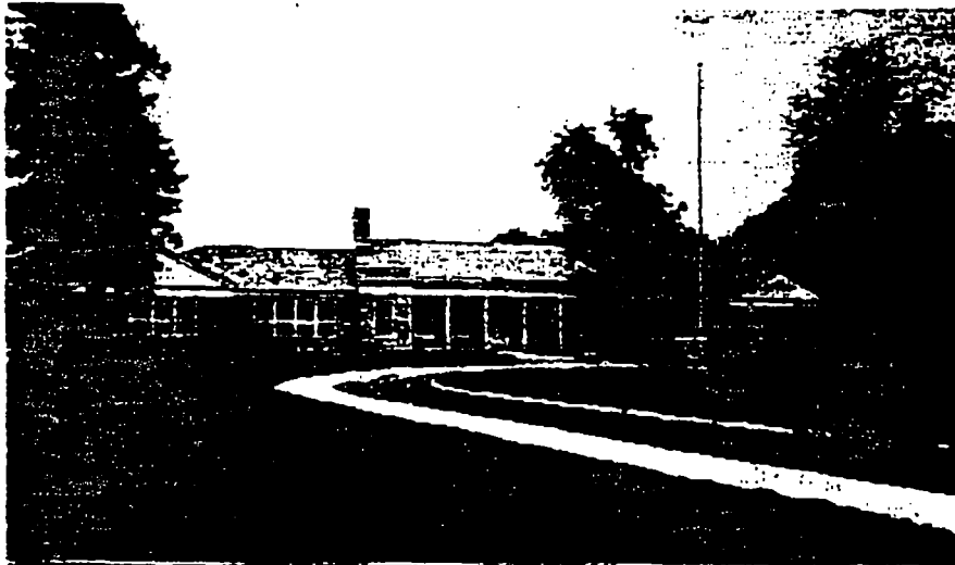
Evans Park Elementary School
