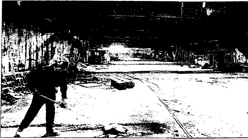
Richie Mckeon sweeps debris at the "Big Dig" tunnel construction project in Boston. The huge undertaking is designed to relieve the city's traffic woes by moving the downtown section of Interstate 93 underground.
