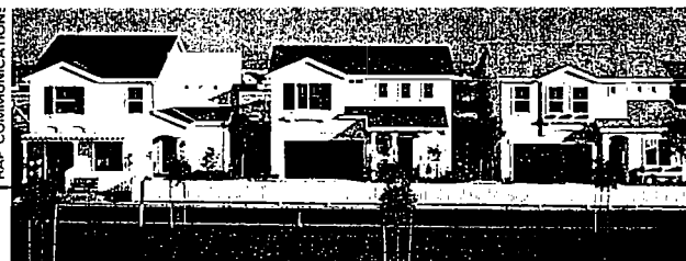
These energy-efficient homes built in Sylmar, California, were constructed as part of DOE's Building America program. The 186 homes include efficient HVAC systems, high performance glazing, advanced framing, and walls with R-19 insulation.
