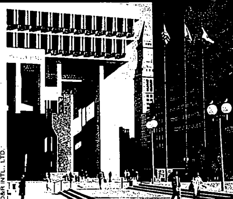
The Rebuild Boston Energy Initiative, a Rebuild America Partnership, has retrofitted more than 8.5 million square feet of building space throughout the City of Boston.
