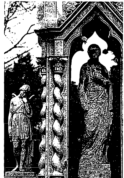
Figure 20. Statues in a Louisville, Kentucky cemetery illustrate the effects of acid rain, created by the reaction between atmospheric moisture and fossil-fuel emissions. A black crust forms on the Madonna because it is sheltered, while the angel has no buildup because of the scouring but nevertheless corrosive action of the rain.
