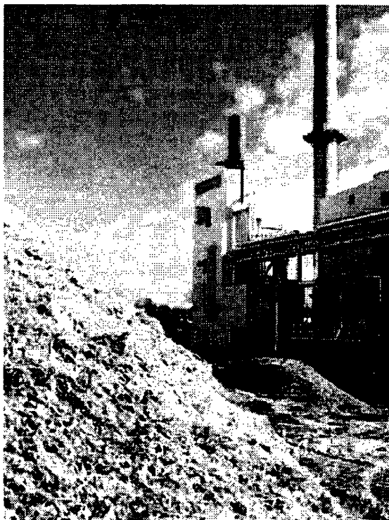
Vermont biomass gasification plant
