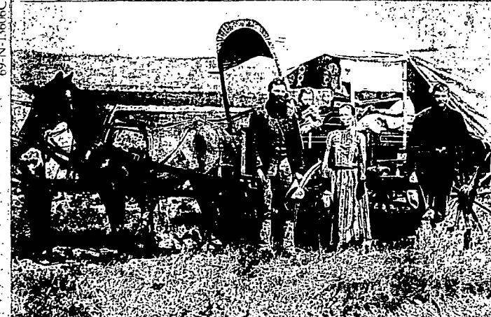
Wagons were rolling west in large numbers in 1886 when this family paused in Loup Valley, NE.
