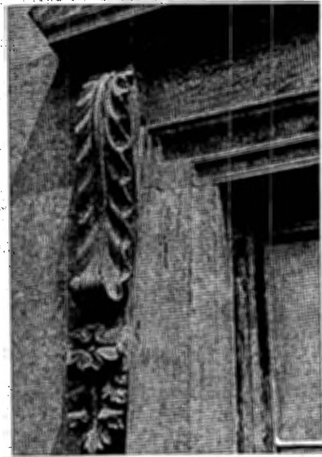
Fig. 17 A typical carved console supporting the first floor window pediments. Note the carved stone moldings that are part of the architraves enframing the windows. photo: Tim Buehner, NPS.
