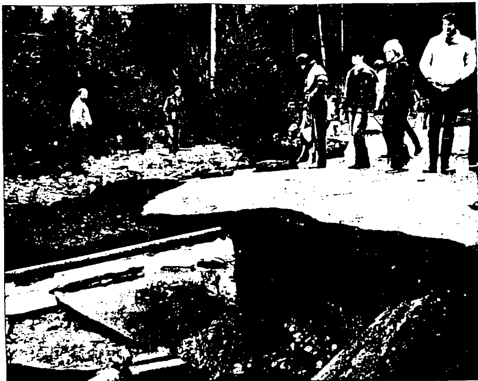
Property losses from floods are not limited to buildings. The ground under this road in Hollywood Hill, Washington, was washed away by torrential rains.
