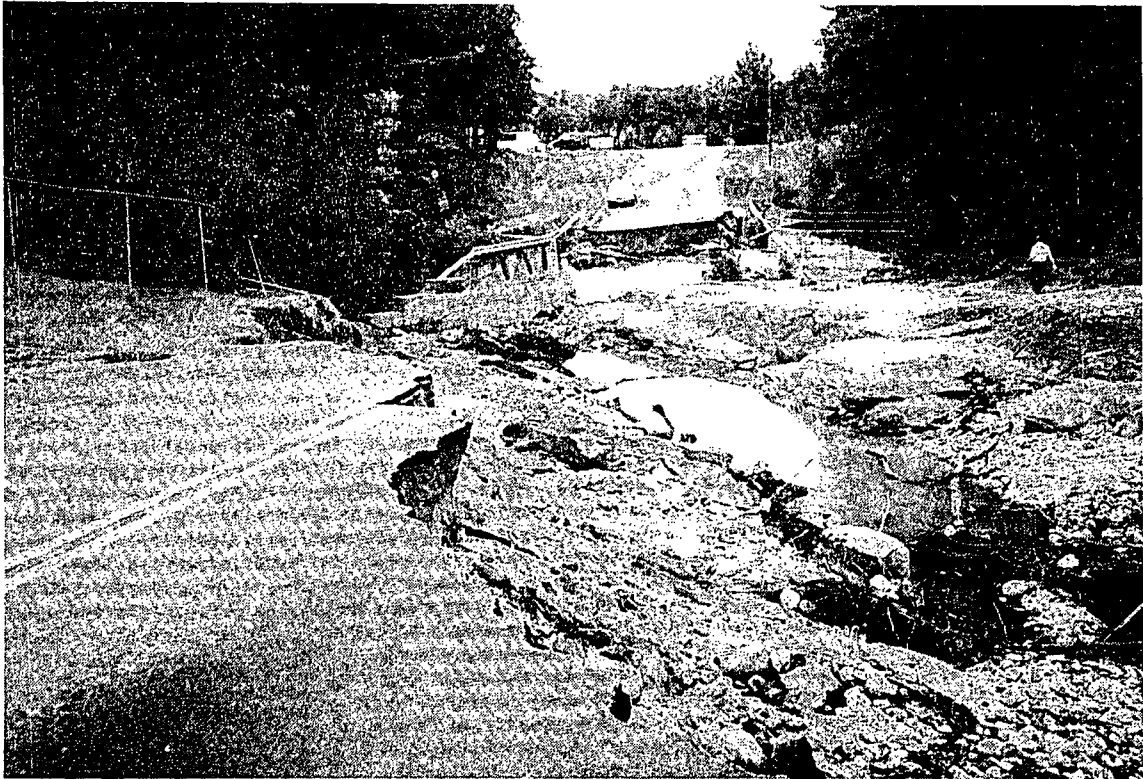
Abutment Failure - Rock Dam, Clark County
