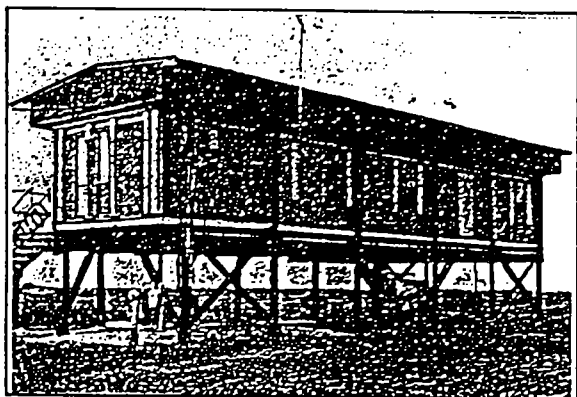
Manufactured Home Showing Cross Bracing and Foundation
