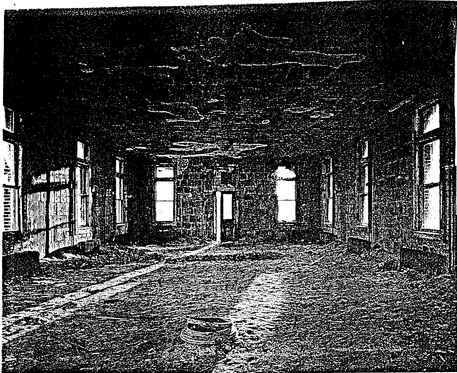
A Hospital Extension This was a ward for women and girls deemed too ill to enter the country immediately. The entire hospital had a capacity of 500 beds. "It is at once a maternity ward and an insane asylum," a long-ago visitor is reported to have said.
