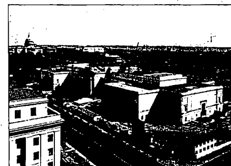
Pope's National Gallery of Art, under construction.
