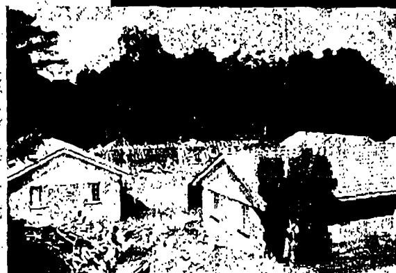
Some of the new houses with the schoolhouse being built in the background.
