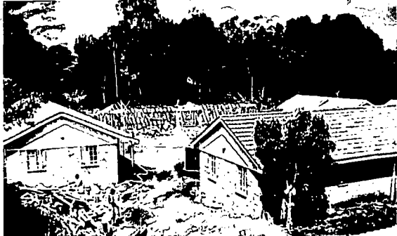
Some of the new houses with the schoolhouse being built in the background.
