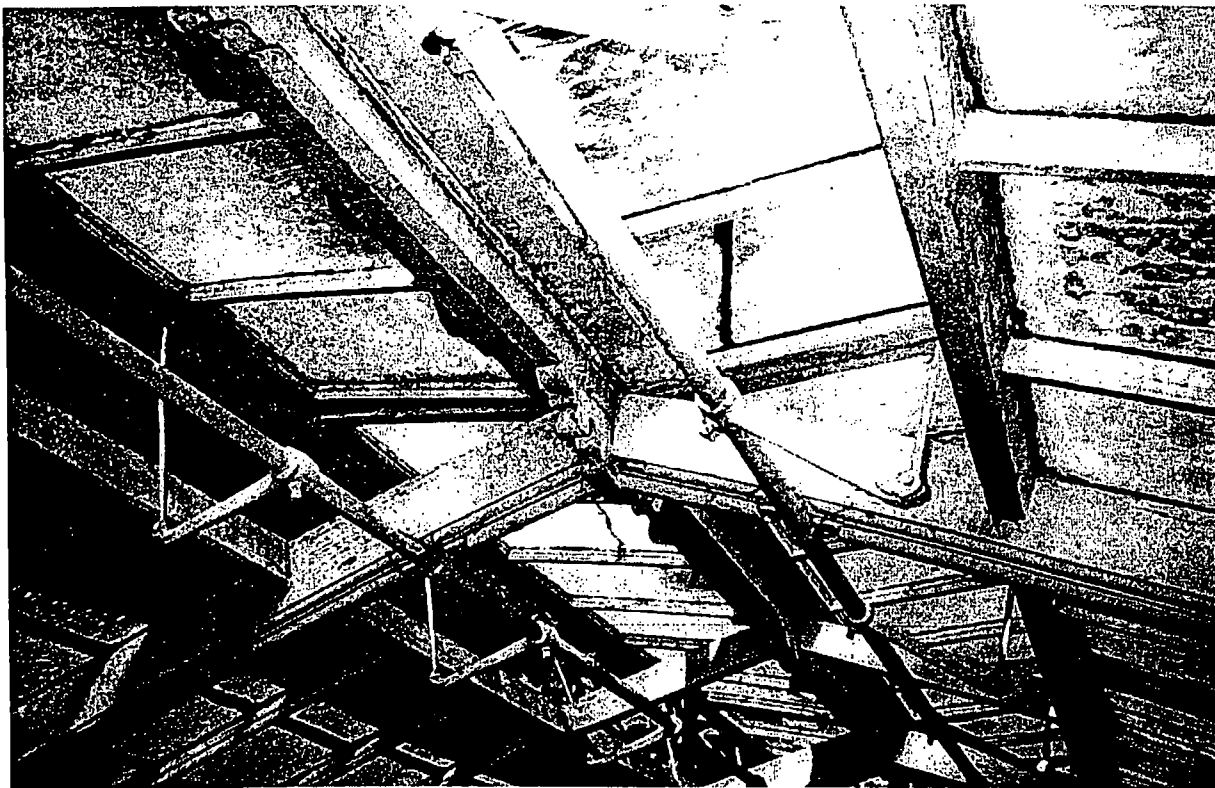
Operable ventilators located on both sides of the ridge beam. Photo source: Architectural Resources Group.
