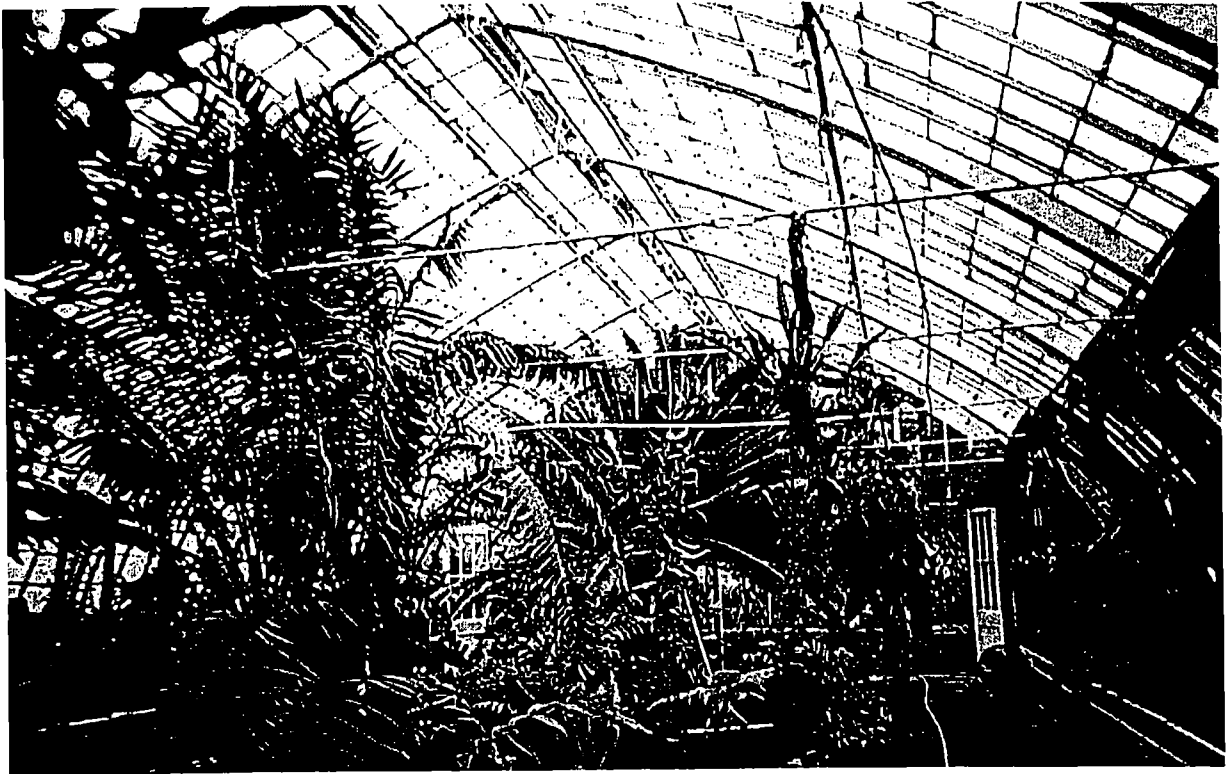
Above: Interior view of the East Wing (Cycad Room). Tudor arches are the predominant form in the structure. Photo source: Architectural Resources Group.
