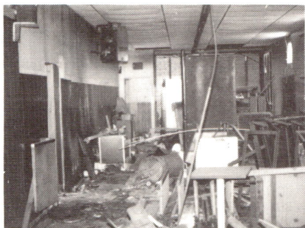
STATE STREET PLAZA, BEFORE RENOVATIONS BEGAN...
