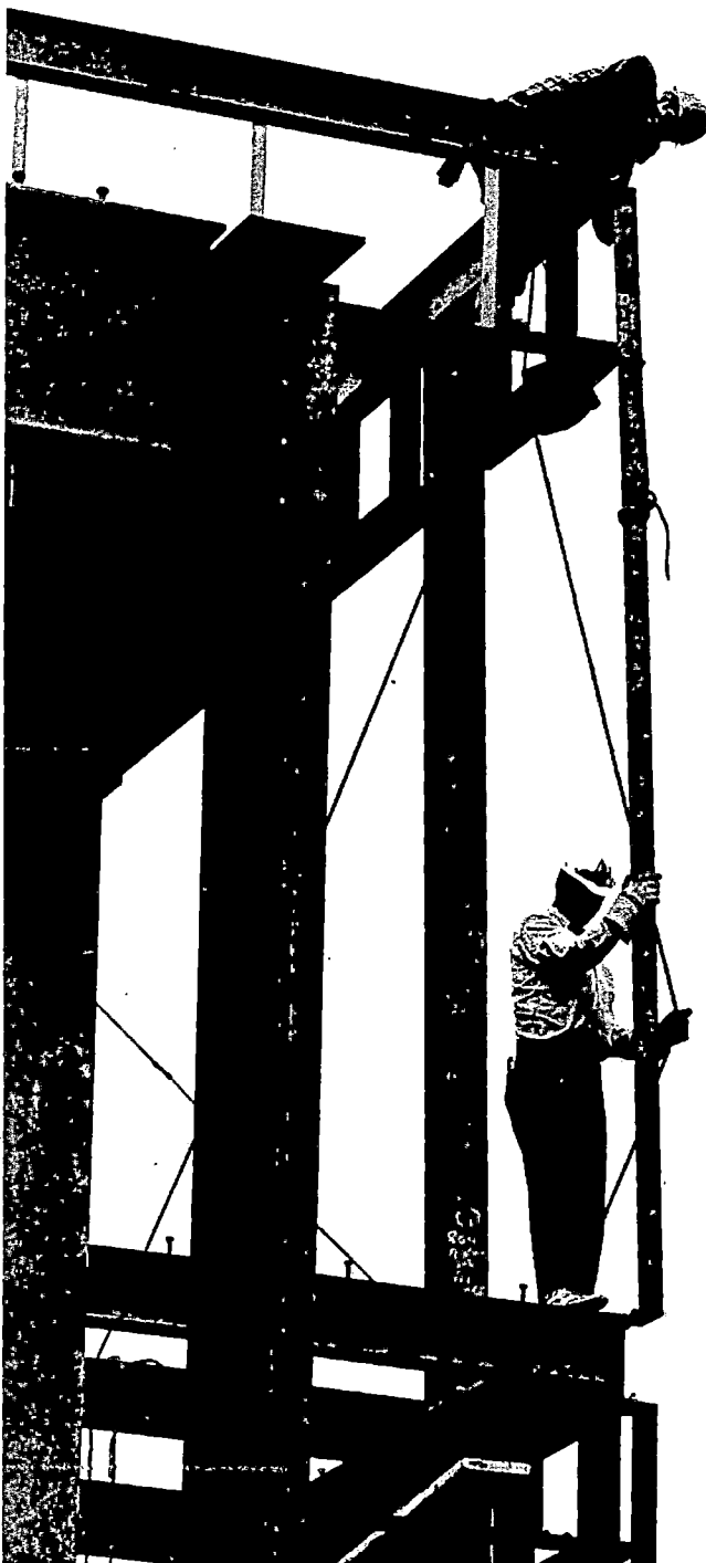
Structural metal workers are among several trades represented in the highest earnings category.
