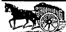
Tons of Broadway dirt, excavated for the Metro by the MTA, will be used in construction of the new stadium grounds at Camden Yards (see Update, p. 2).
