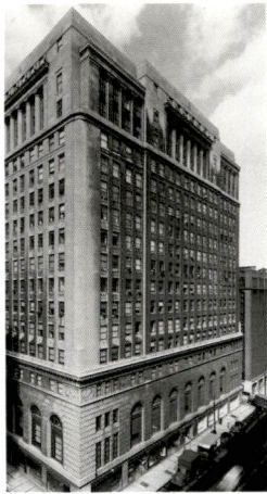
The 14-story Chicago Mercantile Exchange at Washington and Franklin Streets was home to the Exchange for 45 years, 1927–1972.
