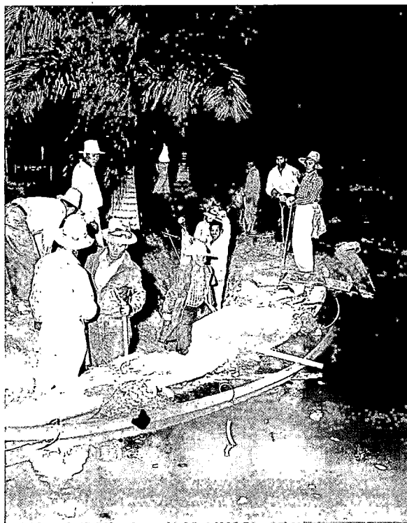
Workers labored into the night of December 7th to repair damage at Hickam Field.
