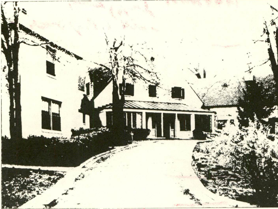
Soon to be demolished to make way for a new $13-million addition, the old wing of the hospital dates back to the 1920s.
