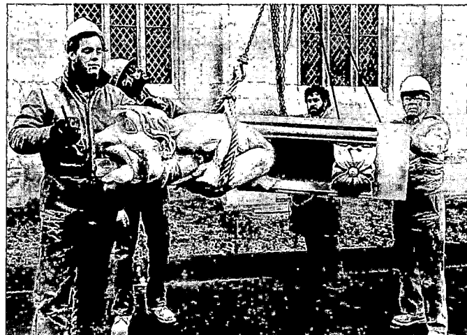
66. The last gargoyle for the cathedral is roped and chained ready for ascent to the top of the tower.
