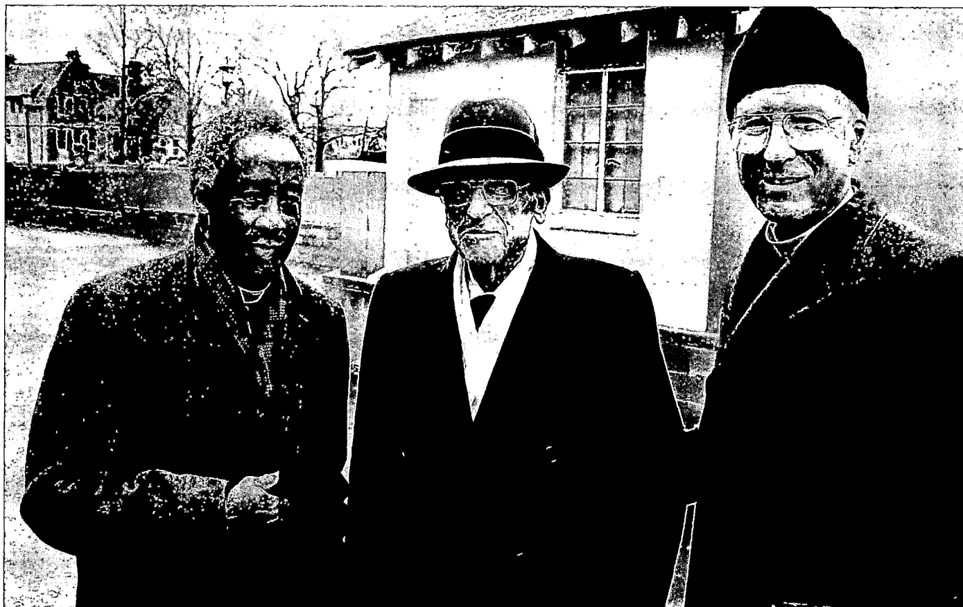
67. Bishop Walker and Provost Perry welcome Dr. Thomas McKnew to watch hoisting of the last gargoyle. Dr. McKnew sang as a choir boy at the setting of the foundation stone in 1907 and was the first on-site construction company superintendent on the cathedral.
