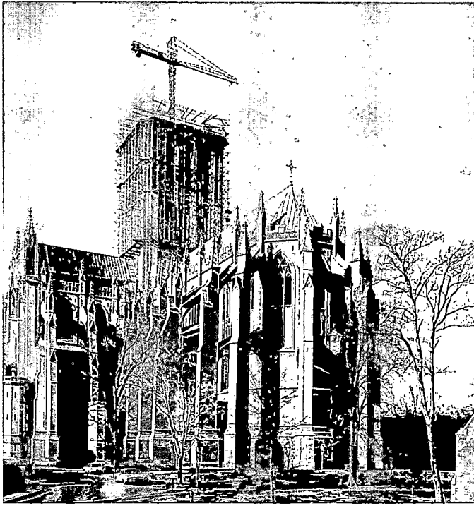
15. The central tower in late 1962 was nearing its roof level.
