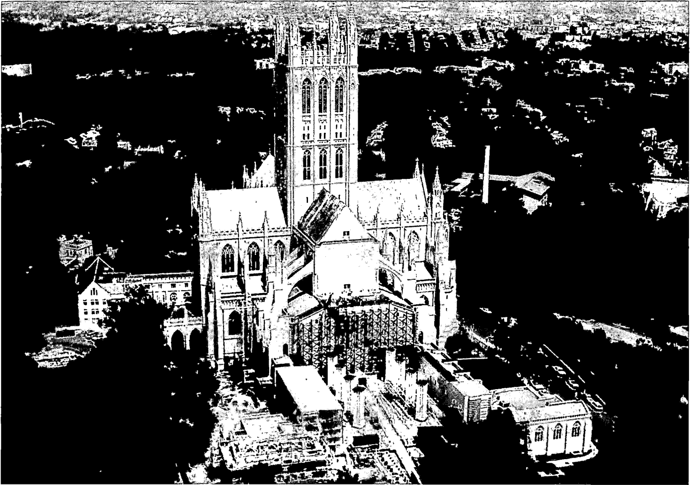
18. In the summer of 1966 the first three bays of the nave are complete and the northwest wing is under construction.
