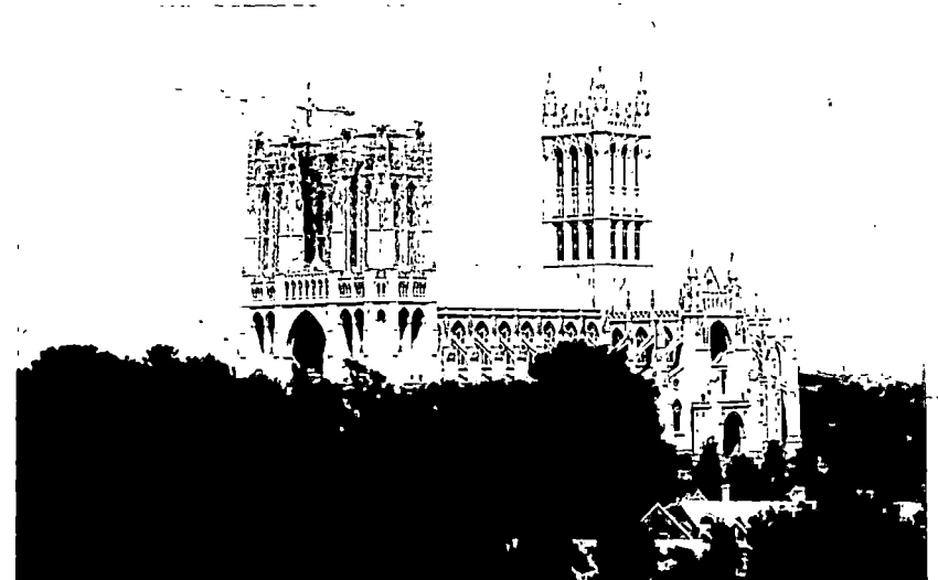
The final stone will be set on Washington National Cathedral on September 29, 1990, culminating a building program that began more than 80 years ago. In anticipation of this event, a year-long series of special events and programs has been planned. Photographer: John Wrigley
