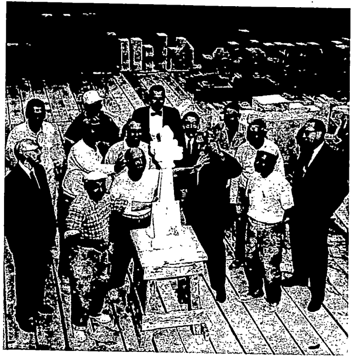
21. Architect Philip Frobman jokingly threatens to destroy the last carved finial for the central tower as stone carvers restrain him.
