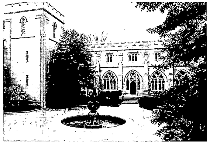
76. The east cloister connecting Bethlehem Chapel and the administration building houses the choir practice room and organists' office on the first floor with offices of the altar guild and clerk of the works on the second floor.
