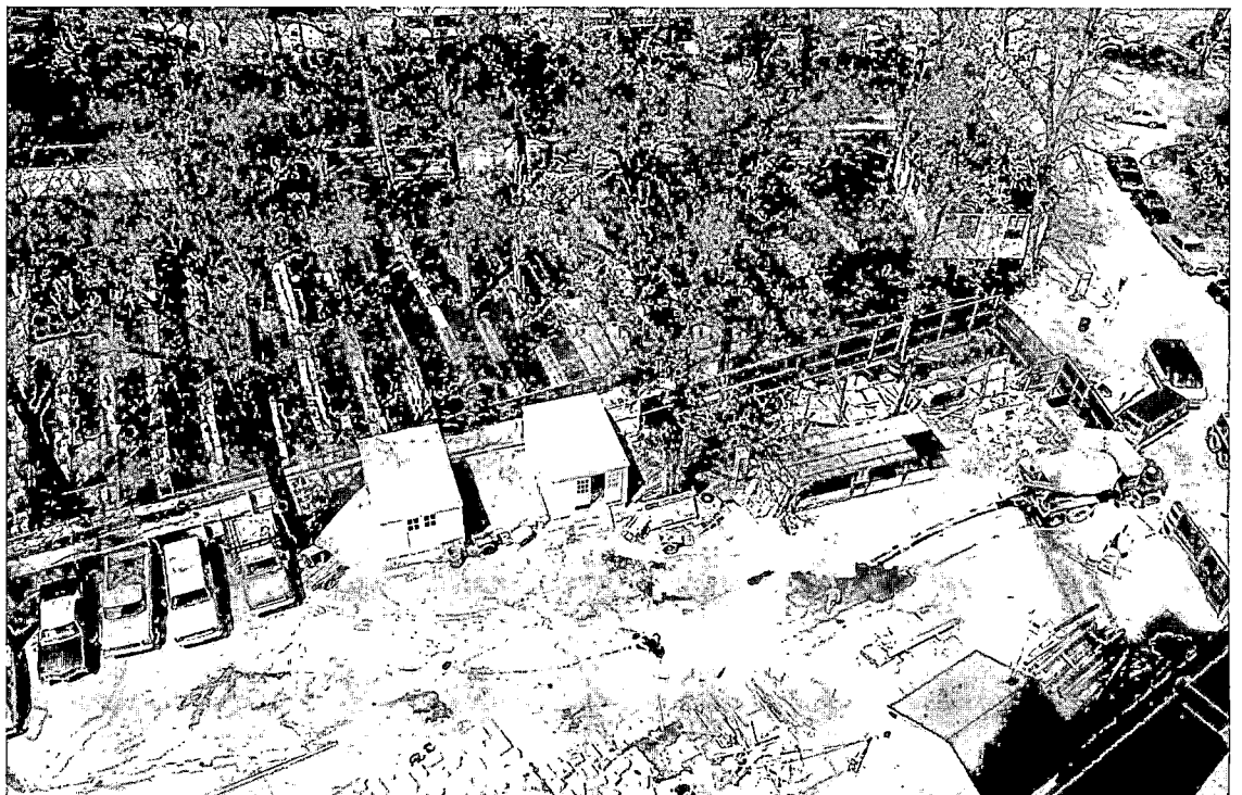
63. The construction yard in all its homeliness. Between it and Wisconsin Avenue are stones awaiting setting.
