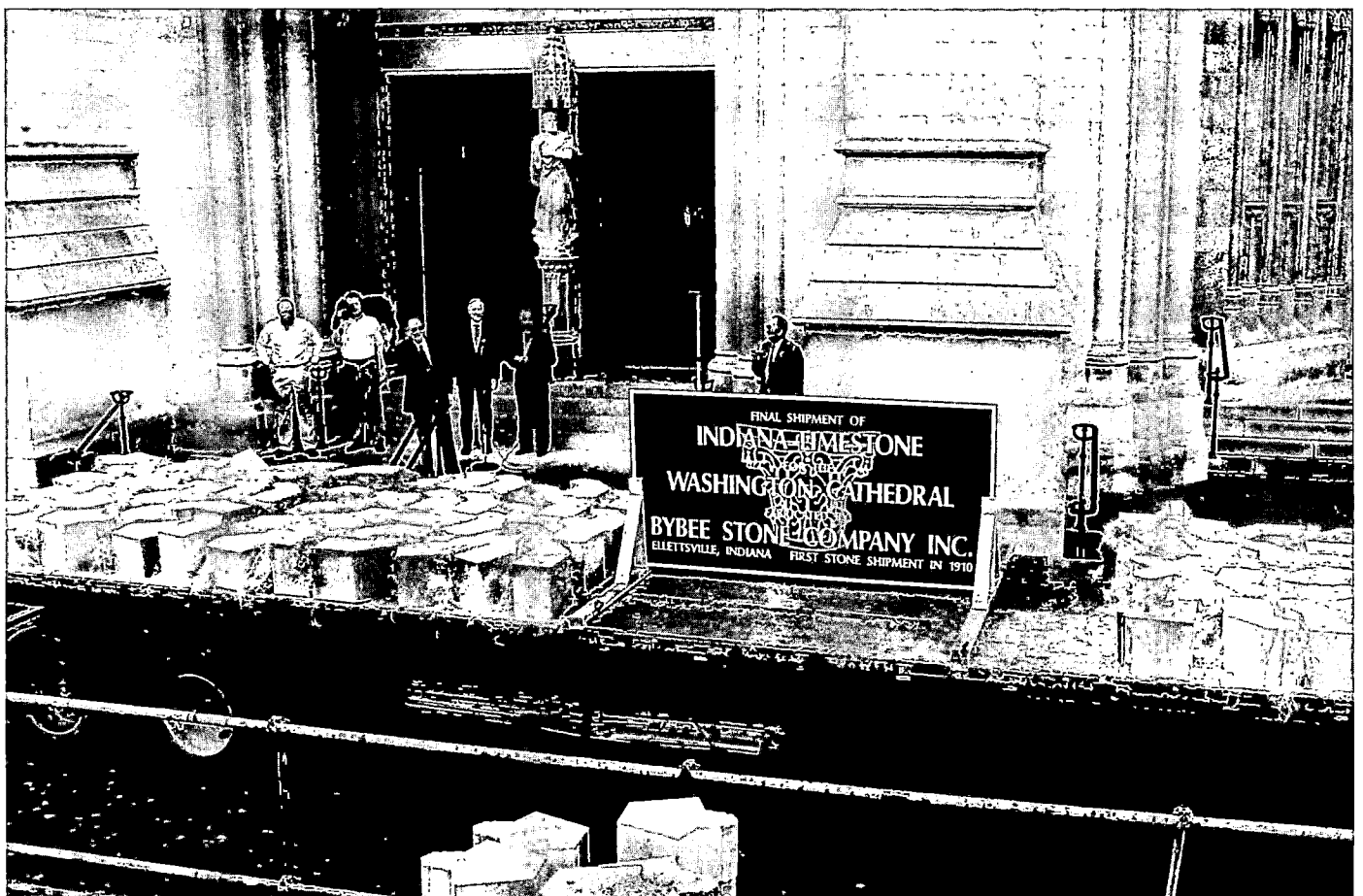
72. After 79 years, the final shipment of Indiana limestone arrived at the cathedral on May 23, 1989.
