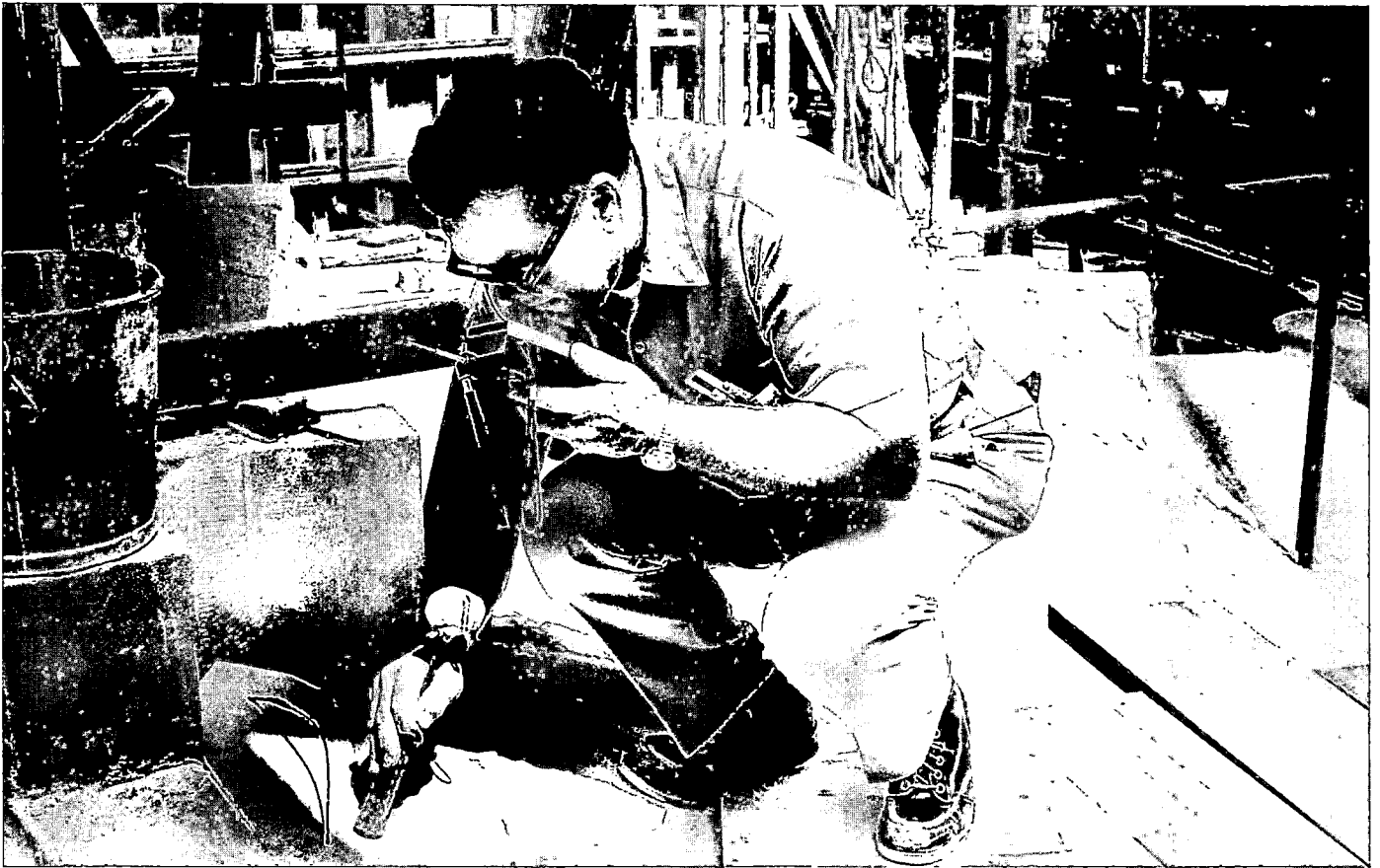
25. Master mason Peter (Billy) Cleland with walkie talkie communicates with the laborer beneath as the last piece of nave vaulting infill closes out the sky forever.
