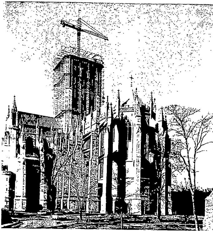
15. The central tower in late 1962 was nearing its roof level.
