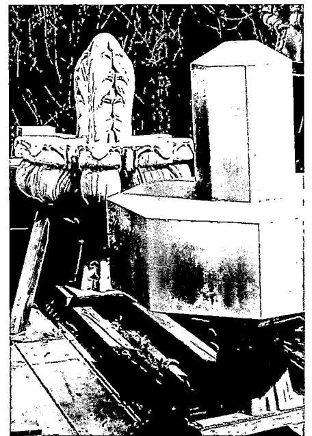
56. In foreground a finial blocked for carving as it arrives from the mill in Indiana. In back the finial after being carved by cathedral stone carvers.
