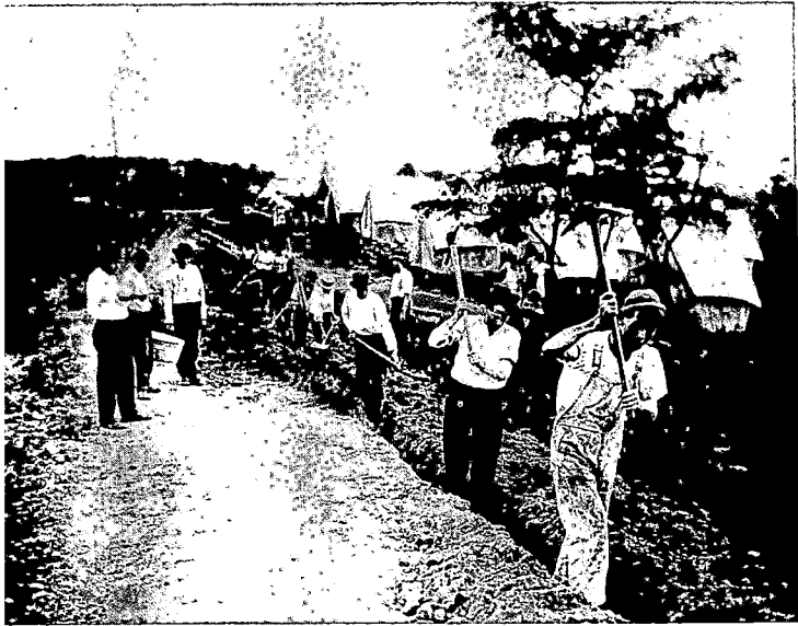
Digging sanitary ditches for the tent city.
