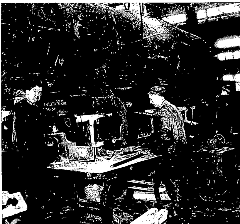
Ed Twomey (left) and his helper, Guy Beeler (right), are grinding boiler checks to fit on a steam freight locomotive in 1935. The workers behind them are using the overhead locomotive crane to support a lever, which they need to set springs and hangers on the locomotive's underframe.
