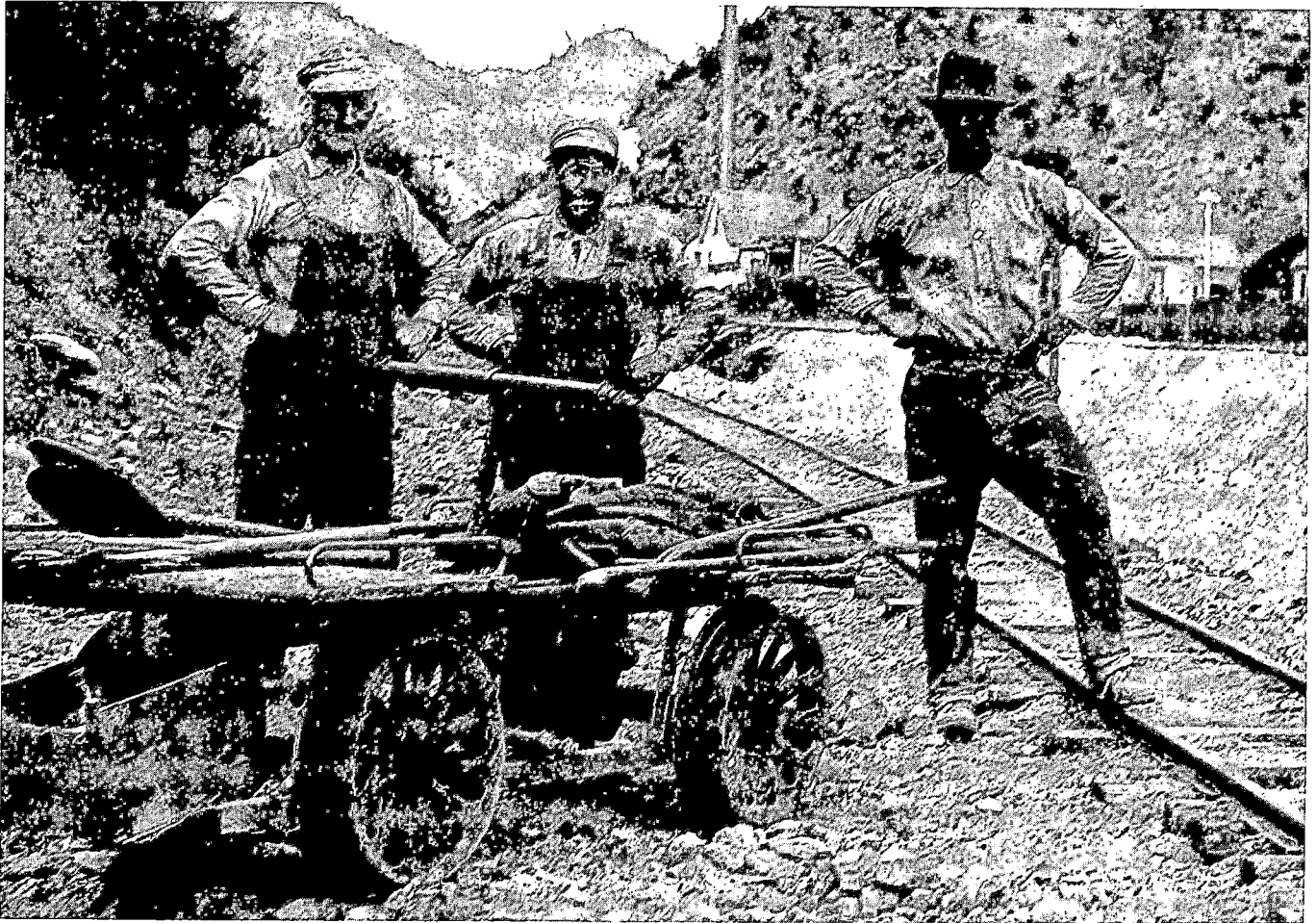
Three workmen stand beside their small maintenance rail car used for mine track repairs, n.d.
