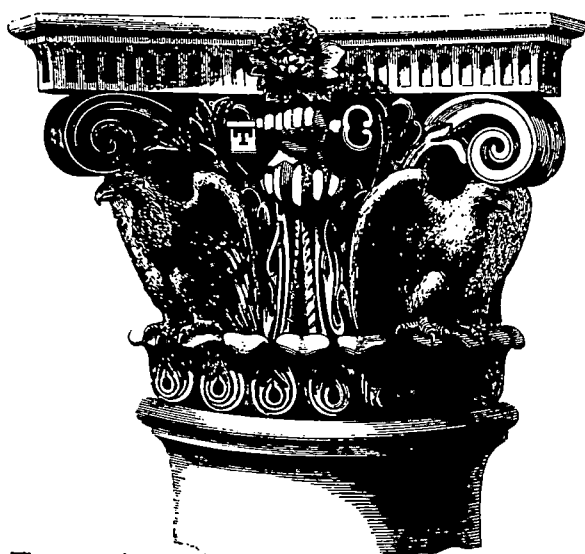
The cast-iron column capitals in the South, West, and North wings are unique to Treasury. They combine elements of Ionic and Corinthian orders of architecture with federal iconography (the gilded eagle and the hand holding a gilded Treasury key).
