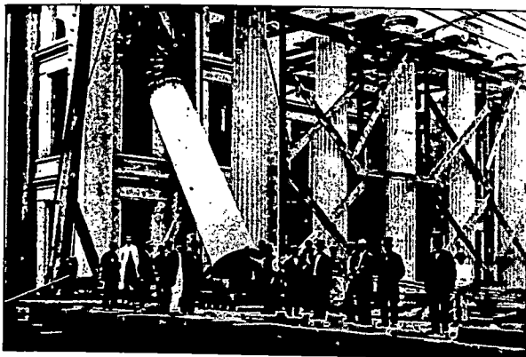
Solid granite columns are hoisted into place on the north portico of the Treasury Building, September 16, 1867. (National Archives)
