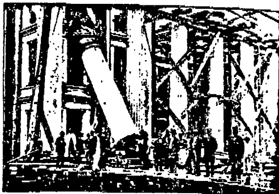
Solid granite columns are hoisted into place on the north portico of the Treasury Building, September 16, 1867. (National Archives)
