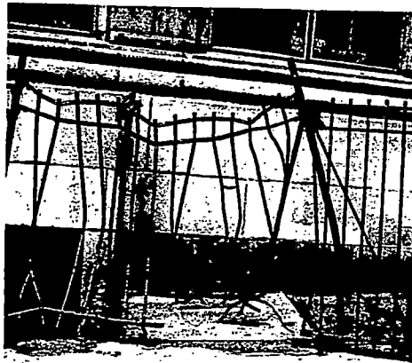
Seward Park's fence, unrepaired for 10 years
