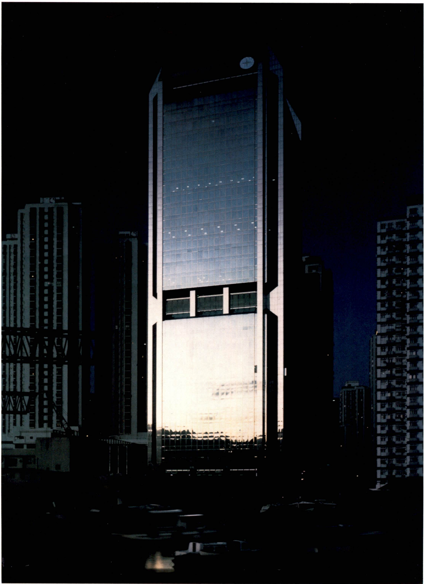
Citibank in Hong Kong, one of the largest office buildings in the world, is furnished with Steelcase products.
