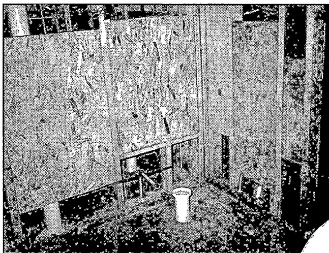
Whole wall reinforcing installed in a Habitat house
