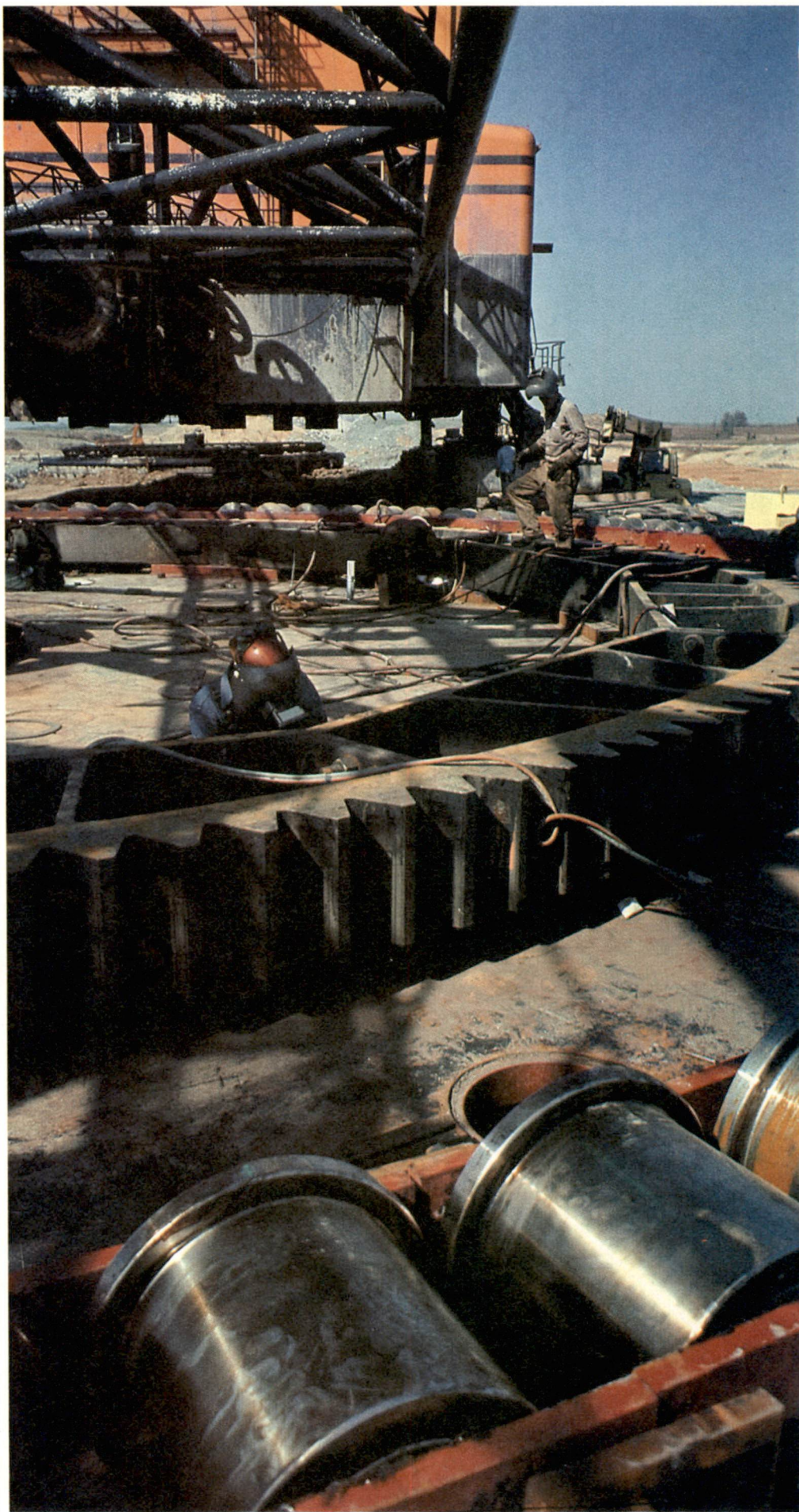
(right) Welders put the finishing touches on the 1.3-million-pound replacement tub. The machine pivots on the rollers—100 of them—around the edge of the structure.
