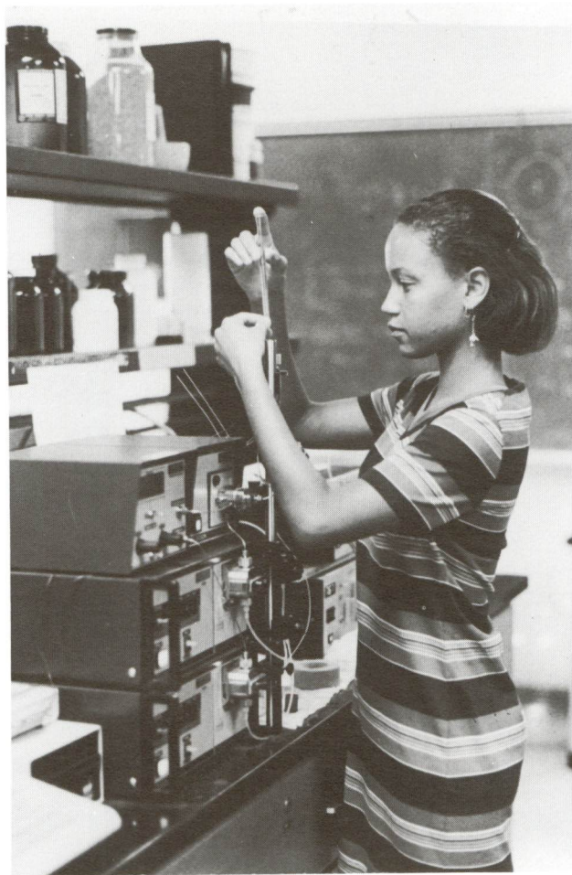
A student analyzes materials extracted from marine organisms using high pressure liquid chromatography. The availability of state of the art instrumentation is critical for training in biotechnology.
