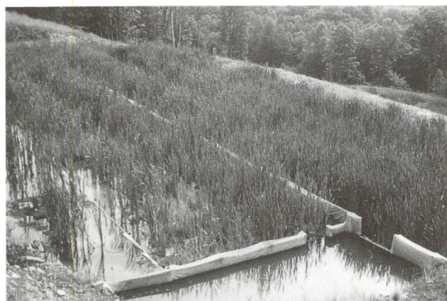
Wetlands constructed on active and abandoned mined sites can be used to treat acid mine drainage. The metals in the drainage are precipitated and/or filtered by the wetland and microorganisms.
