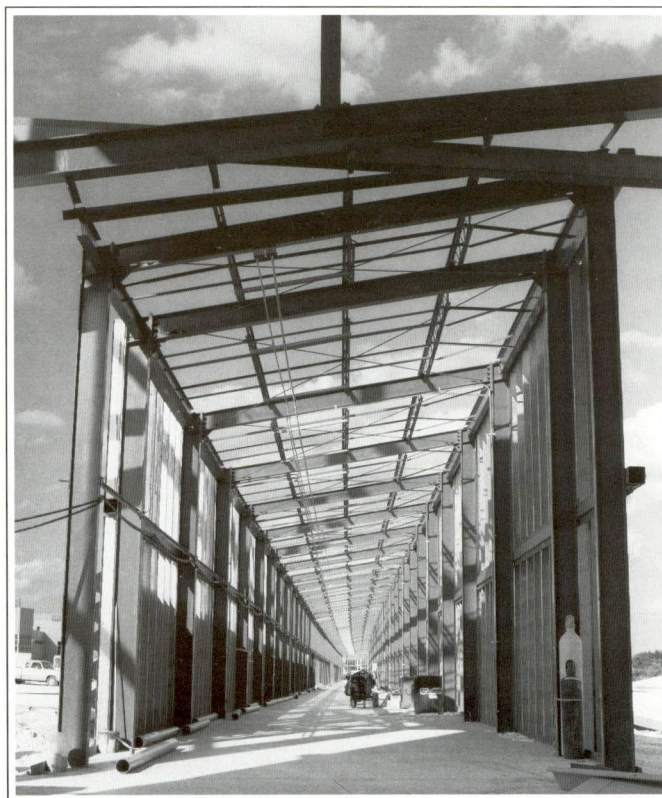
The building for the Accelerator System String Test (ASST) during an early stage of its construction, which was completed in 1991.
