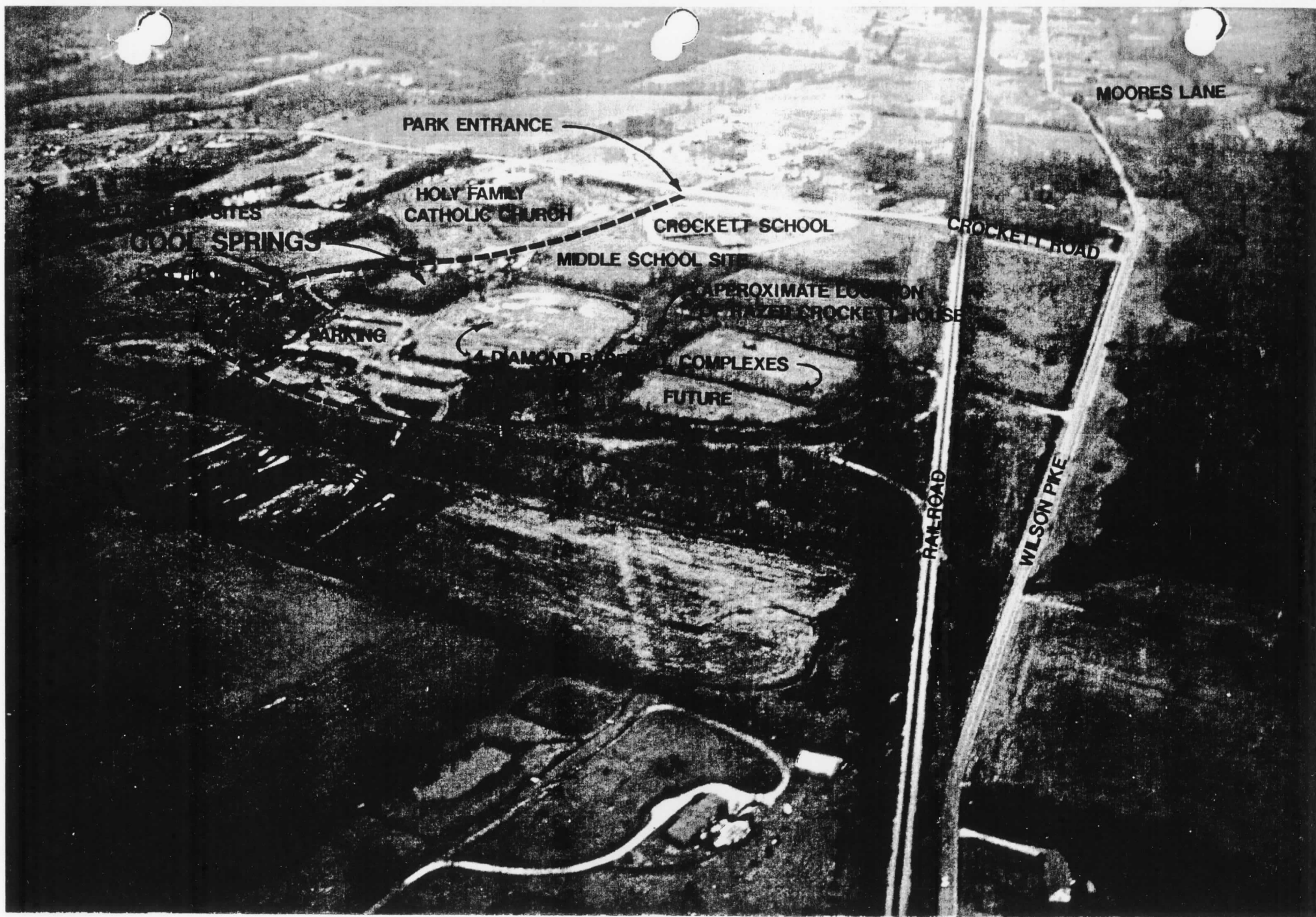
AERIAL VIEW OF CROCKETT PARK
