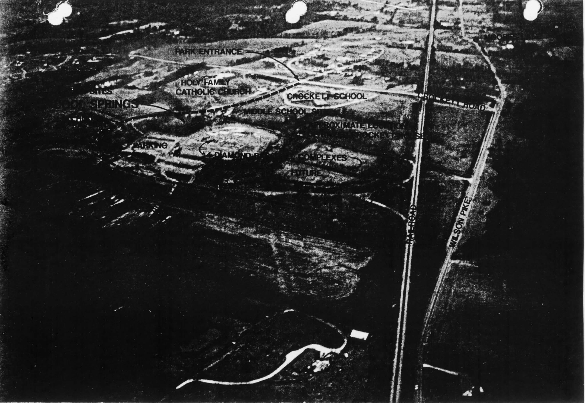
AERIAL VIEW OF CROCKETT PARK
