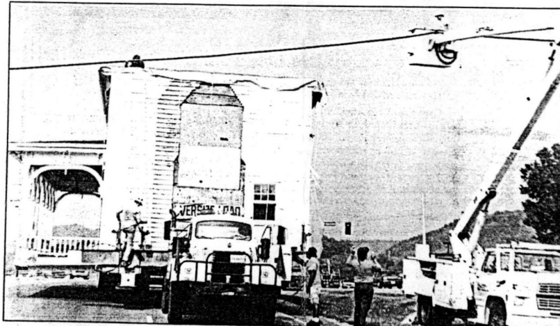
Above and at right: Stansell electric company employees lift lines along Moores Lane so that the Cool Springs farmhouse can pass underneath. The house is being moved by W.P. Camp and Sons, who are third generation housemovers. Barring rain, the second portion of the house will be moved Wednesday from Mallory Lane through the mall area to Moores Lane, Wilson Pike, through Oak Hall and Somerset subdivisions to Crockett
