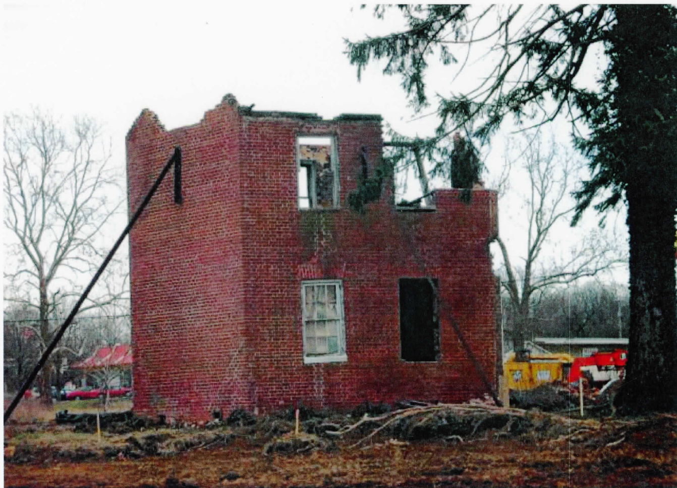
GENOWINE-NICHOLS-COLLINS HSE DURING DEMOLITION JAN 2008
